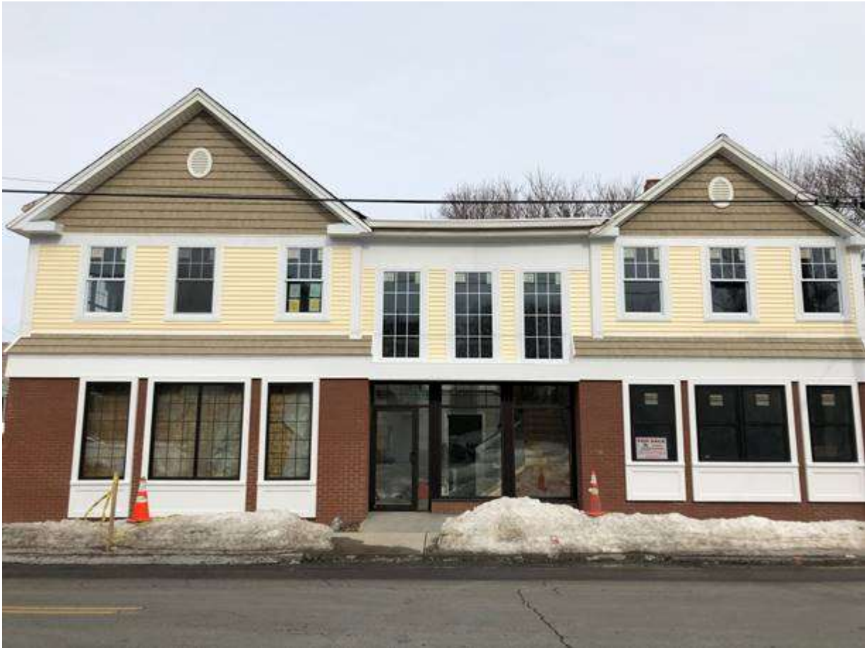
839 Eastern Avenue after
